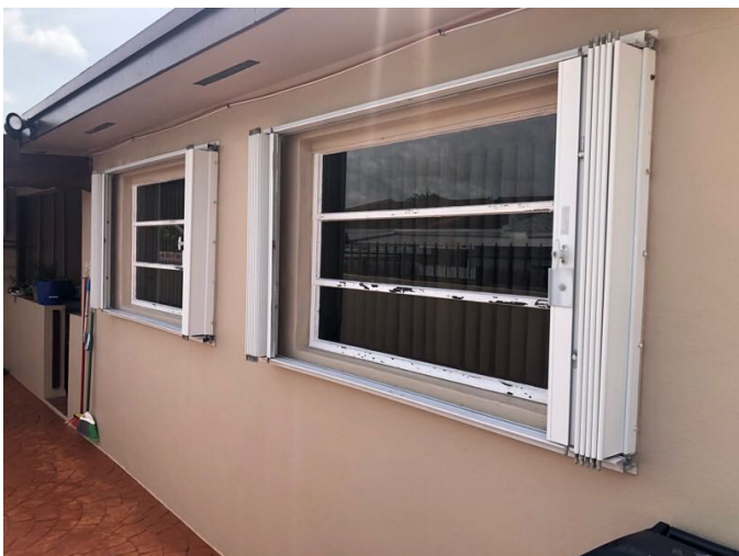
Protected windows showing accordion shutters
