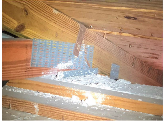
Roof to wall attachment (single wraps)
