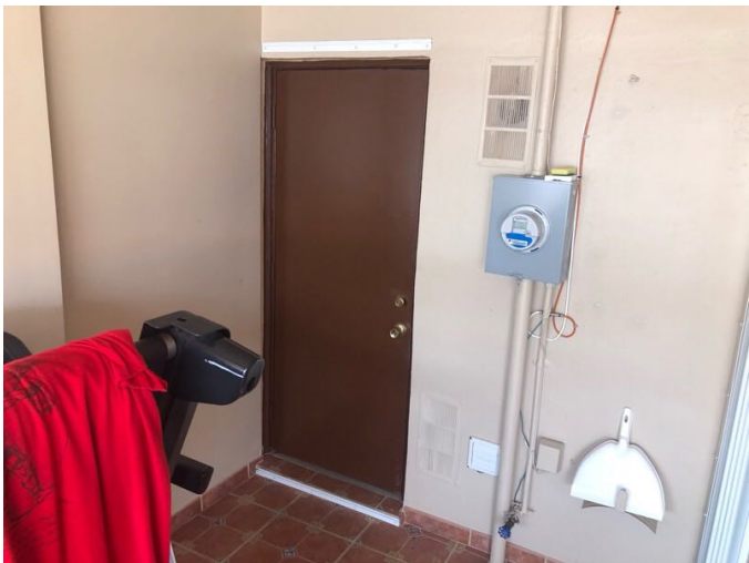
Protected door showing tracks
