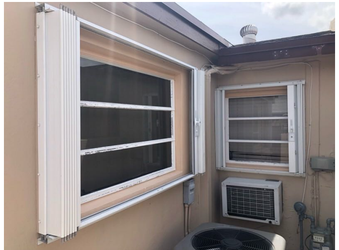
Protected windows showing accordion shutters
