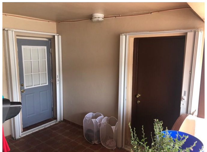
Protected doors showing accordion shutters
