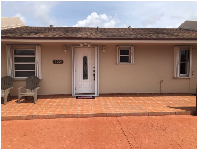
Protected windows and doors showing accordion shutters
