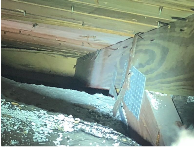
Roof to wall attachment (single wraps)
