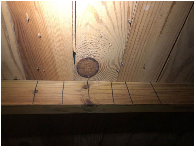
Roof deck attachment ( 2 per board)
